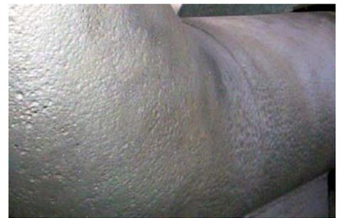
The adjacent photo shows a very clean surface and is ready to paint. The corrosion has been thoroughly removed even from the steel pits. The surface is thoroughly dry and has little or no flash rusting.
